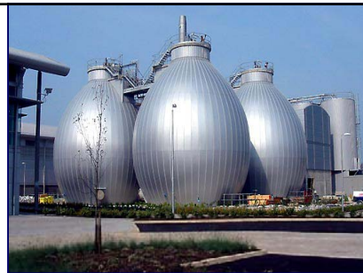
Picture of a typical egg-shaped sludge reactor
